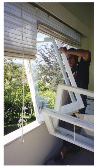
Dismantle good-quality building parts carefully for reuse on your project or for resale (Ward Demolition).
