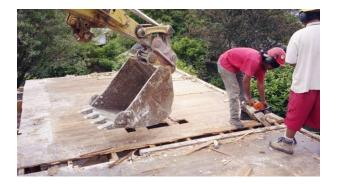
Ward Demolition removing wooden floor boards from a house and salvaging the timber.
