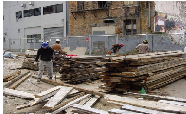
Stacking timber according to dimensions at Northern Roller Mills deconstruction.
