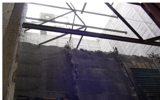
Steel beams and concrete panels can be recycled (Ward Demolition).
