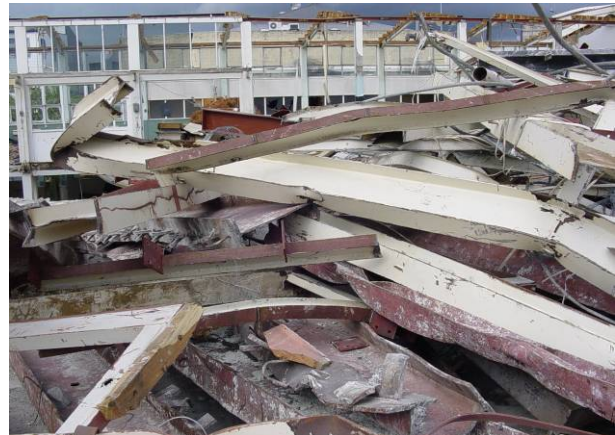
Metal sorted for recycling (Ward Demolition).
