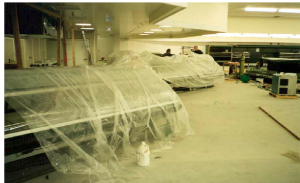
Soft plastic waste is common at fit-out stage (Hawkins Construction).
