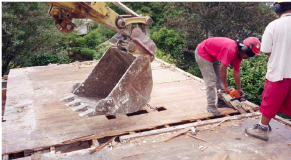
Salvaging floor boards (Ward Demolition).
