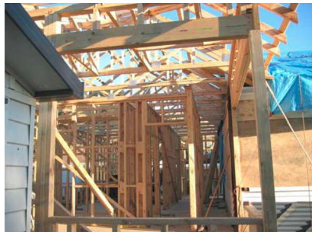
Prefabricated framing saves timber off-cuts on site.
