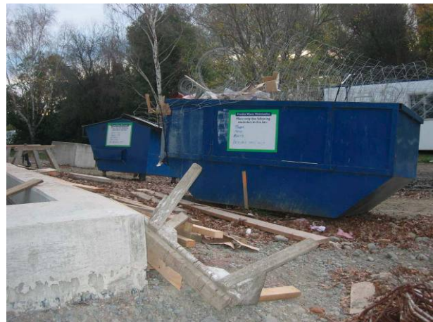
At South City Library, Mainzeal chose a contractor who sorted recyclables off site. One skip was for landfill waste and the other for all recyclable waste.
